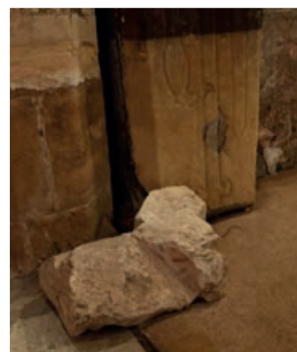
The highest 20th century flood
